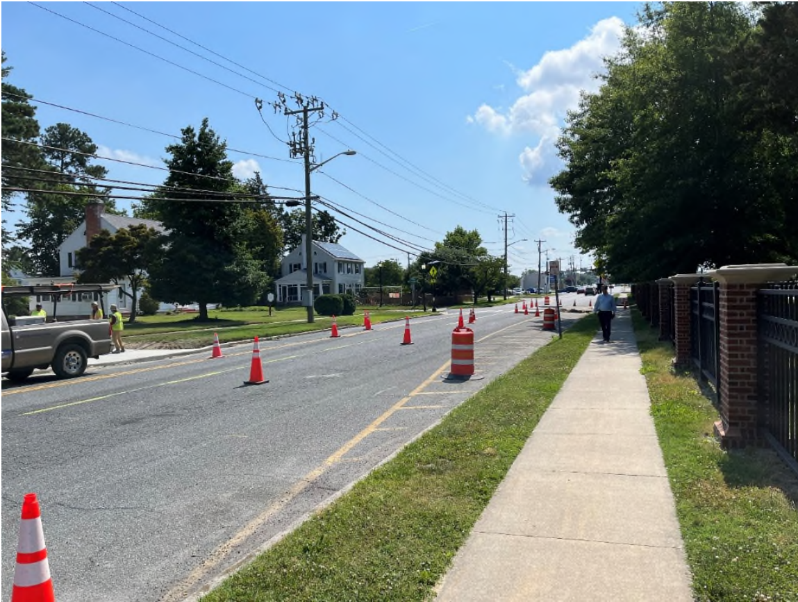
Figure 3: W College Ave Cycle Track Construction
