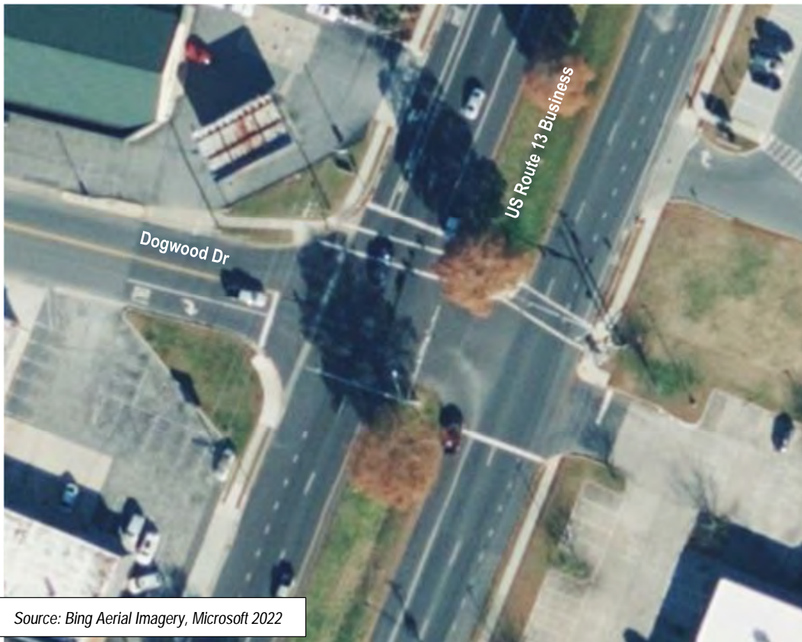
Figure 5: US Route 13 Business and Dogwood Drive
