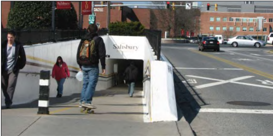
Heavily used pedestrian underpass at Salisbury University
